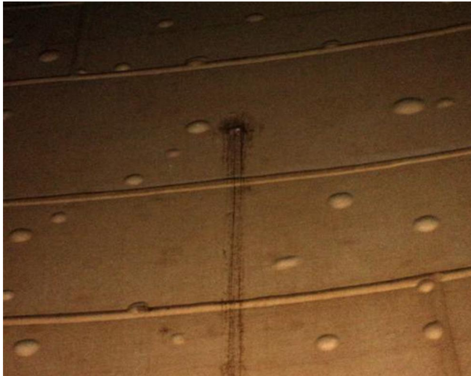
Bubbles in rubber lining
