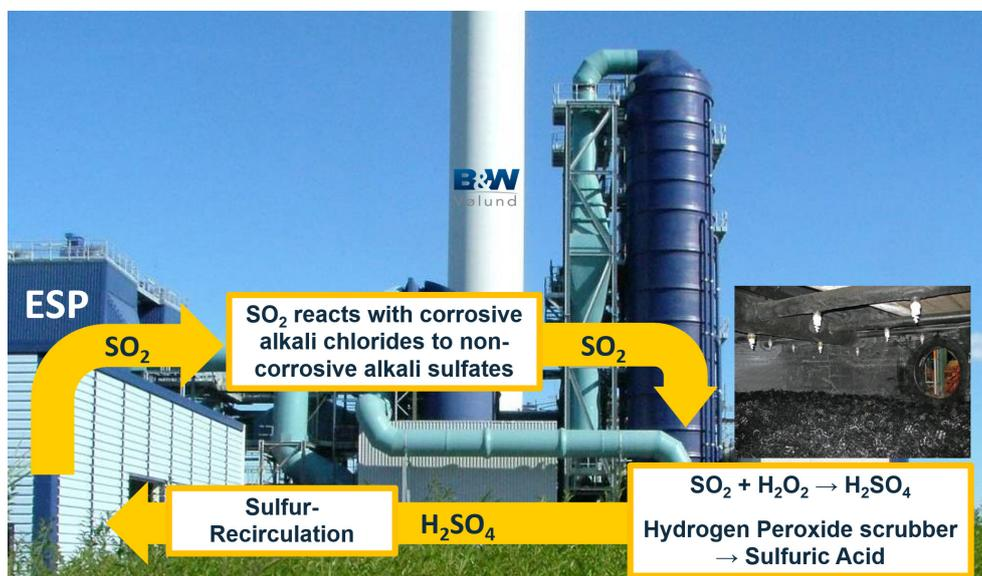
Figure 5: The flue gas treatment is seen together with the main chemical reactions.  $\text{SO}_2$  is captured in the wet scrubber using  $\text{H}_2\text{O}_2$  to produce  $\text{H}_2\text{SO}_4$ . The  $\text{SO}_2$  concentration can now be maintained at a higher level, by dosing sulfuric acid into the furnace, which enables the alkali chloride to react to non-corrosive alkali sulfates.
