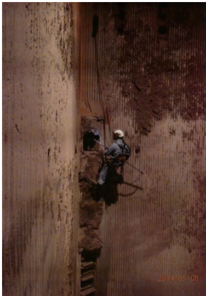
Figure 1. Cleaning of the furnace walls performed at Västhamnsverken.
