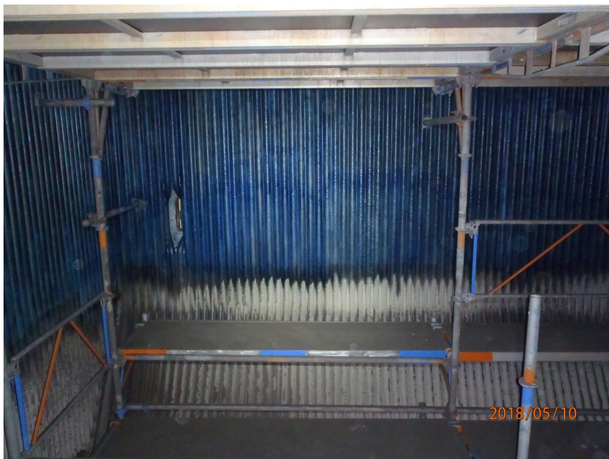
Figure 145. The west wall of the lower part of the furnace after it was cleaned and recoated in 2018.
