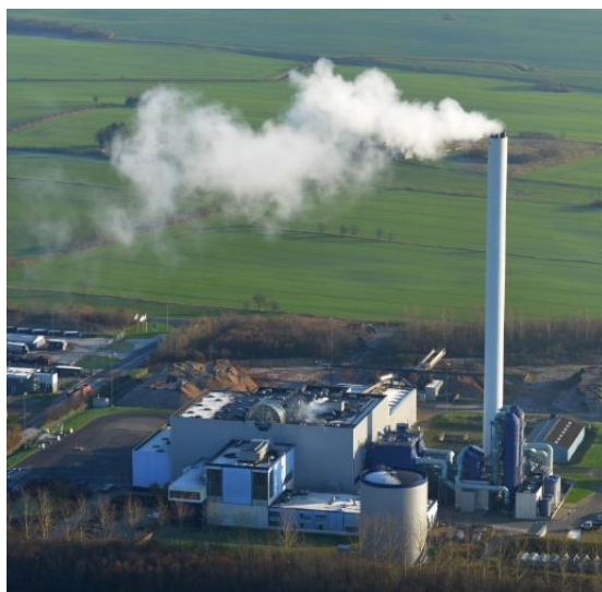
Figure 3. Maabjergværket biomass and waste fired power plant
