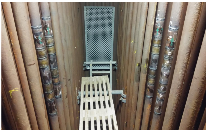
Figure 9. Test materials welded into the superheaters of MEC Waste-to-Energy boiler K1. Superheater 2B is to the right and superheater 1B2 is to the left. The gas flows from the right to the left.
