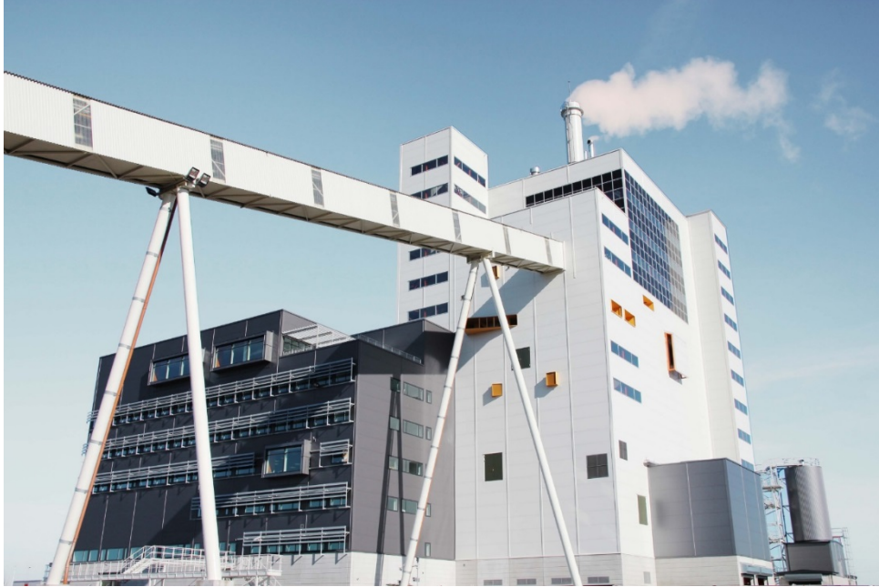
Figure 6. CHP plant Örtoftaverket.
