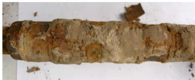
Figure 120. Online corrosion probe after the test campaign 2.
