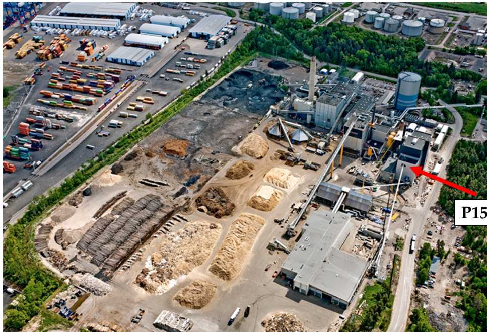
Figure 1. Overview of the Händelö plant, Norrköping
