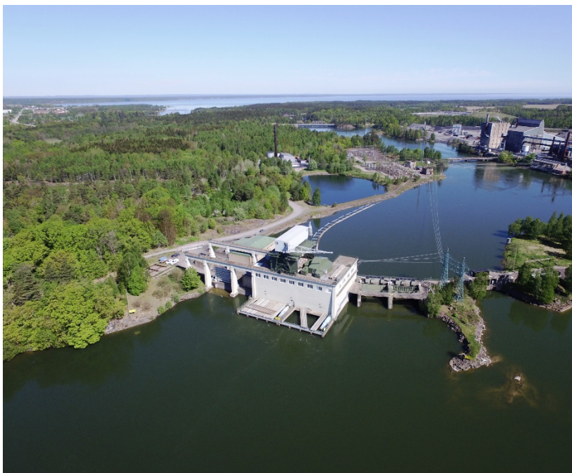
Figure 2 Power plant in Göta älv. Photo Norconsult.
