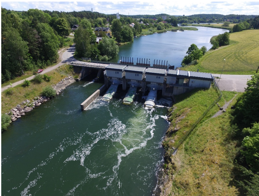
Figure 3 Aerial photo Motala ström. Photo: Norconsult.
