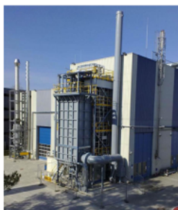
Pilot plant, Linde AG
