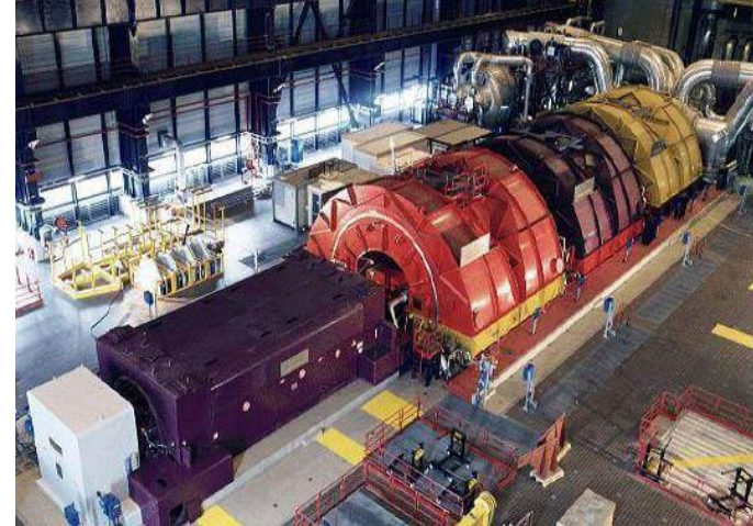
A large scale turbine equipped with HP/IP, 3 LPs and generator
