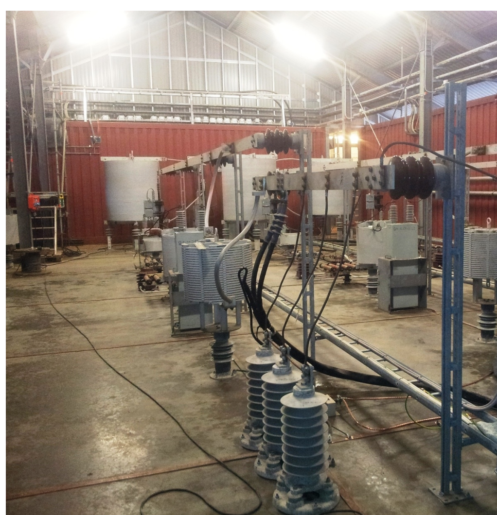
Big Glenn 4 MW wind turbine and the 8 MW HVDC-VSC station with filters and surge arresters
