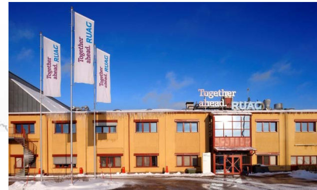
Linköping Mechanical systems
