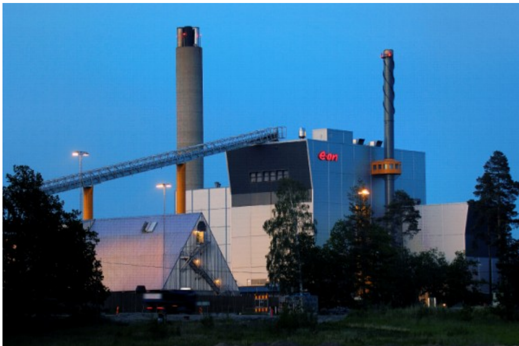
Figure 2. The waste incinerator plant P14 at Händelöverket
