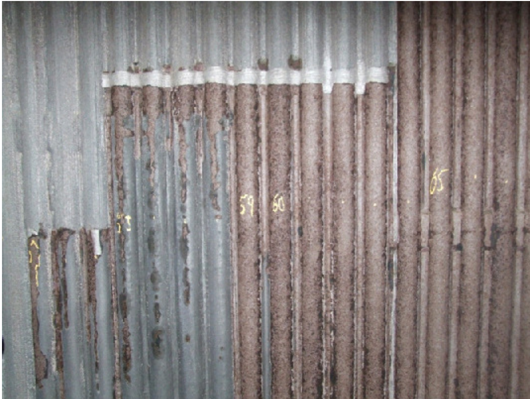
Figure 4 Waterwalls after sand blasting
