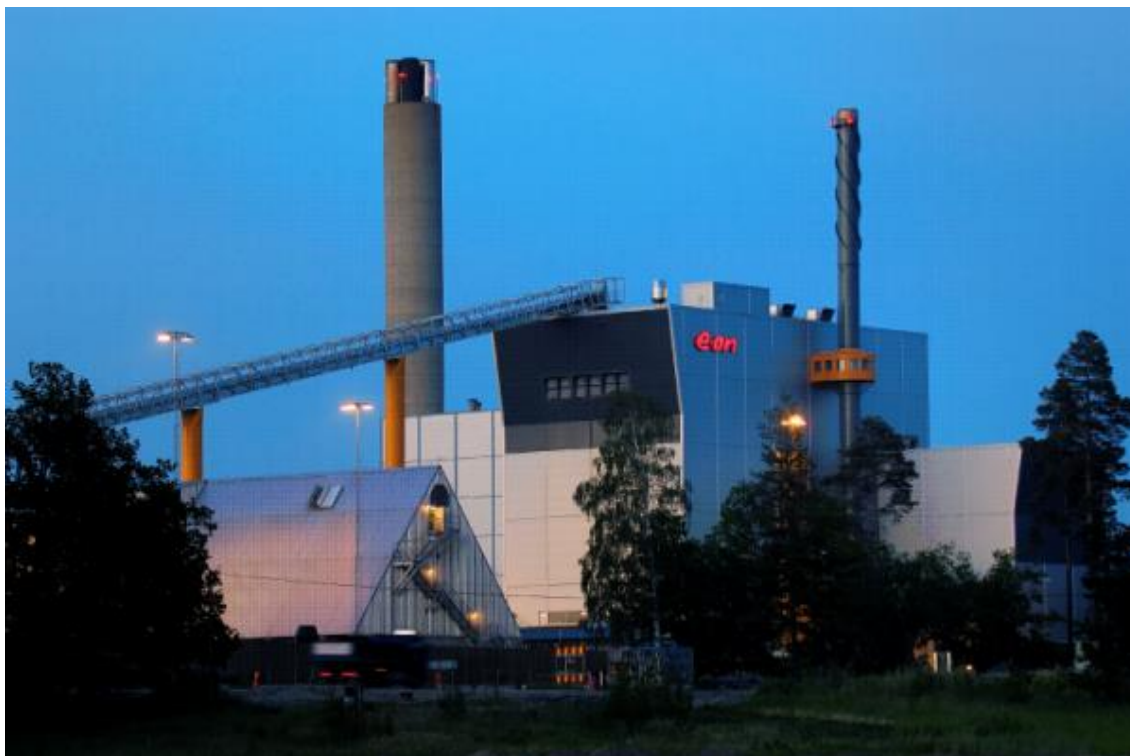
Figure 5-1. The waste incinerator plant P14 at Händelöverket.
