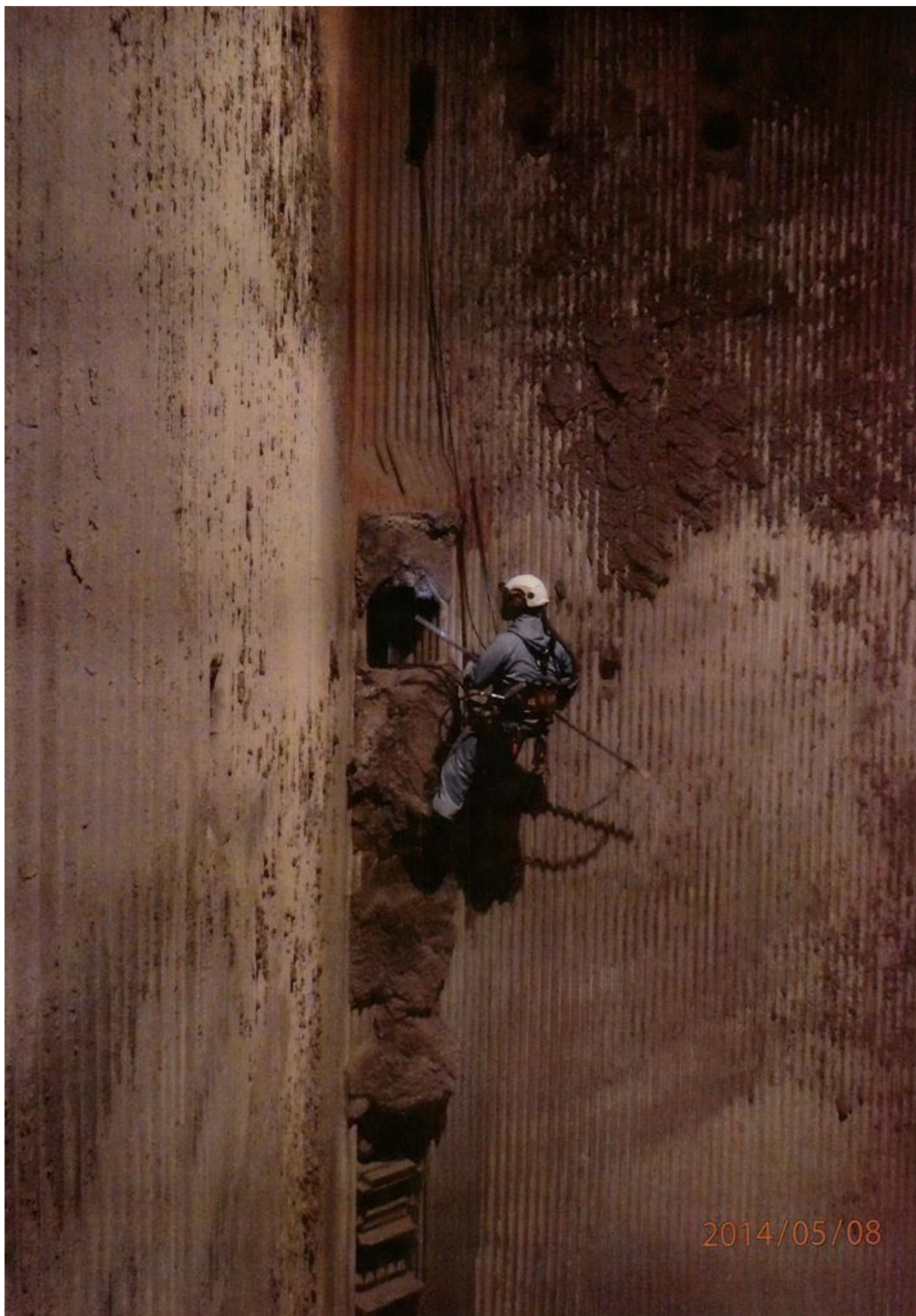
Photo 1. Cleaning of furnace wall fouling at Västhamnsverket
