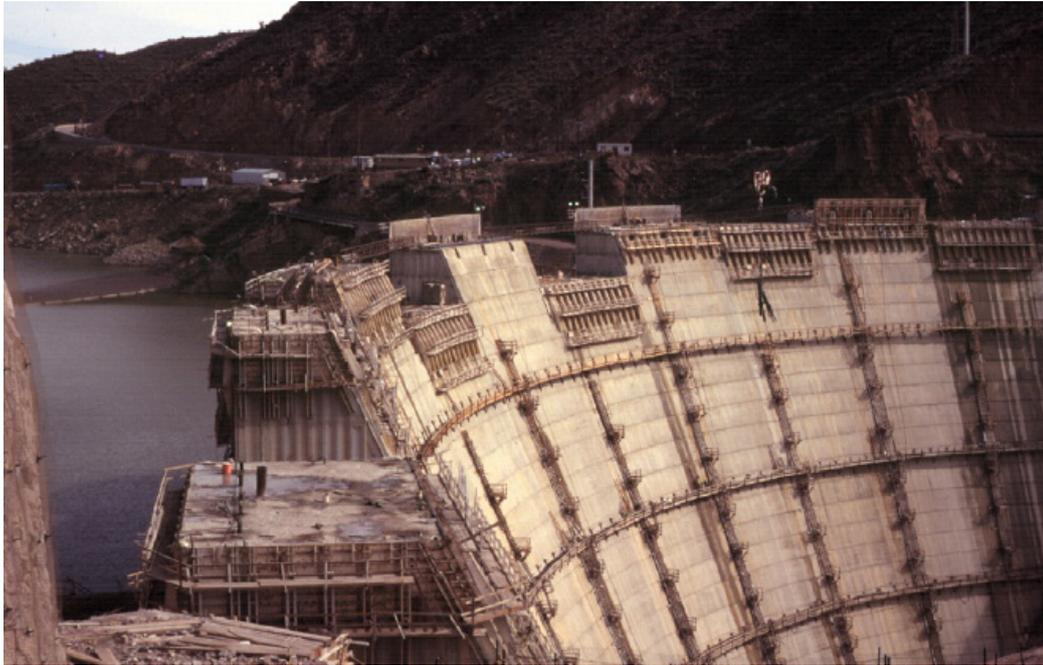
Figure 6-9 Construction of an arch dam where the shear keys of the contraction joints are visible, from James and Dollar (2003).
