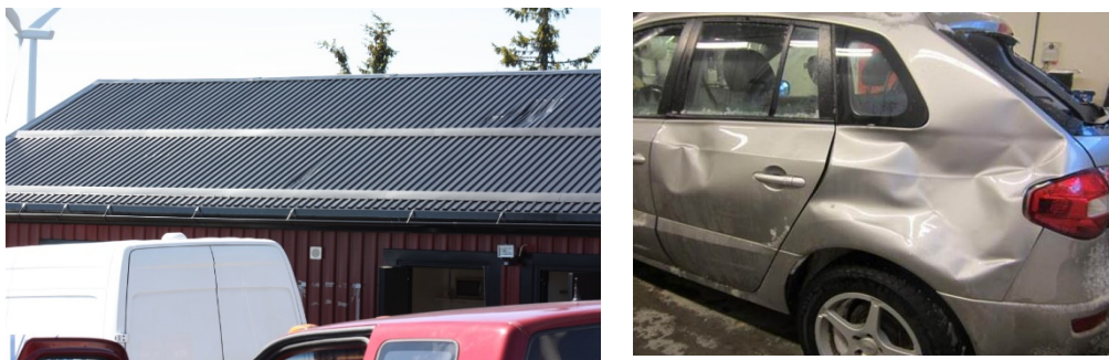
Figure 17. Damage to the roof of the building and the car, caused by ice throw on the site
