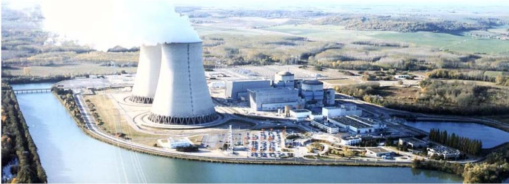
**Fig. 4. Nuclear power plant at the Nogent-sur-Seine site, where two PWRs (1 300 MW each) with their cooling towers to the left are operating.**
