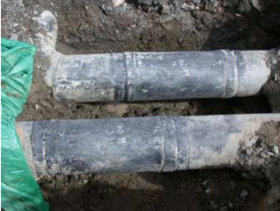
Figur 4.6 Frilagda skarvar vid Gustaf Melins gata. Excavated joints at Gustaf Melins gata.
