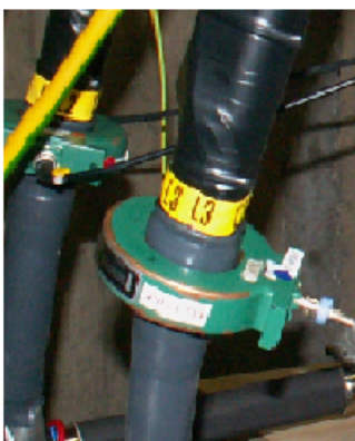
Figure 18: Current monitor Pearson Type D 101 (photo left) and the parameters
