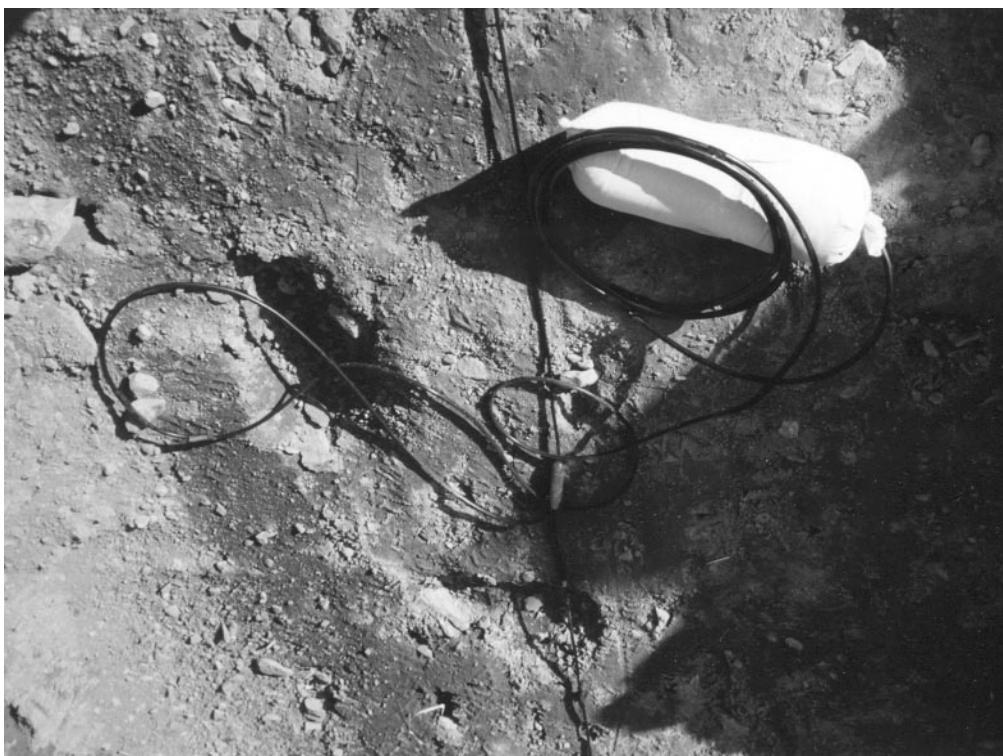
Figure 4 SP-electrode to be buried on the crest of the dam core.
