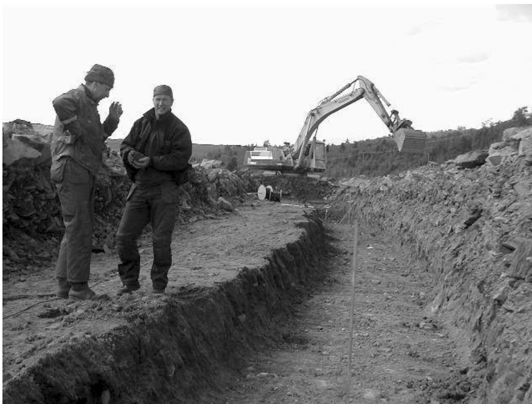
Figure 11 Installations at Sädva.
