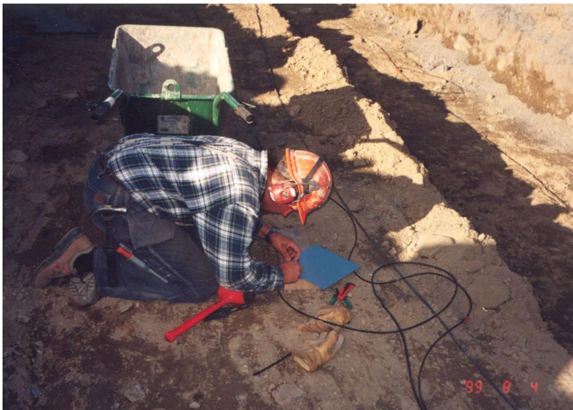
Figure 3-4: Installation of resistivity monitoring electrodes and cables.
