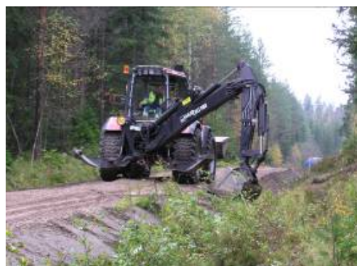
Figur 4: Ökad bärförmåga, minskad tjälproblematik, grus- och skogsbilvägar. Figure 4: Increased stability and reduced frost and thaw related problems for gravel roads and roads for forestry.
