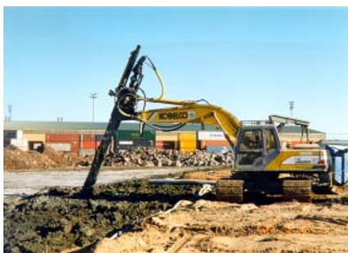
Figur 5: Stabilisering av lösa jordar, terrass & muddermassor, markexploatering. Figure 5: Stabilization of soft soils, subgrade, sediments, development of land.
