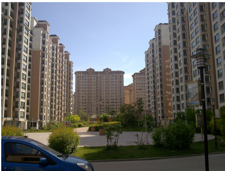
Picture 13. Part of the new residential area connected to the visited substation.
