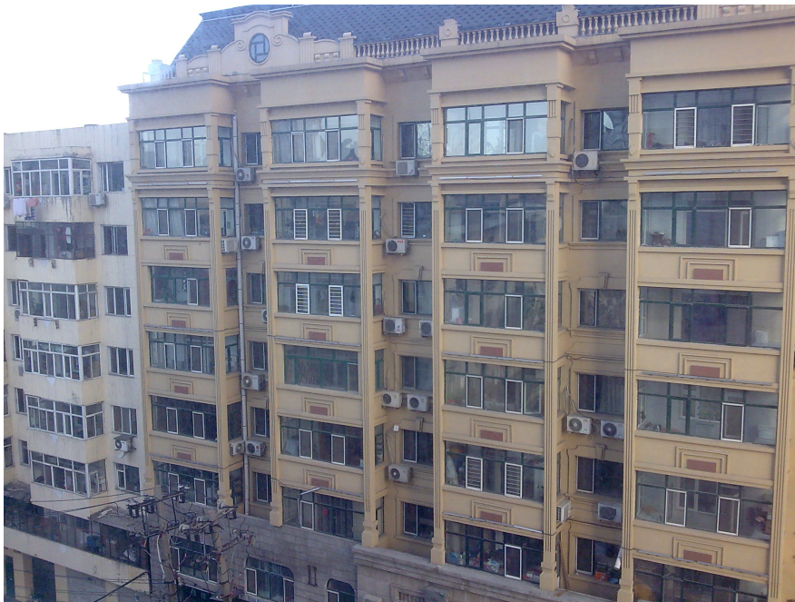
Picture 3. The high penetration of room air-conditioners (RAC) in China illustrated by a residential building in central Harbin.
