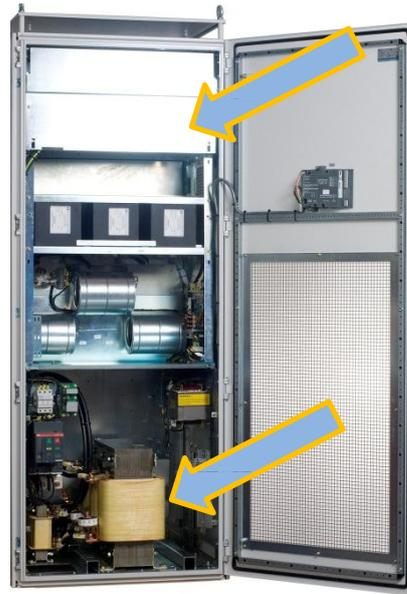
**Figure 22** The circuitry responsible for the high currents and magnetic fields may be located in this panel.
