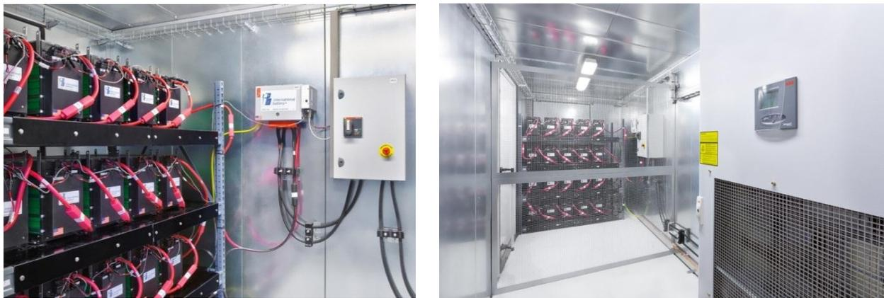
**Figure 3b** Left: battery storage room; right: view from the control room.
