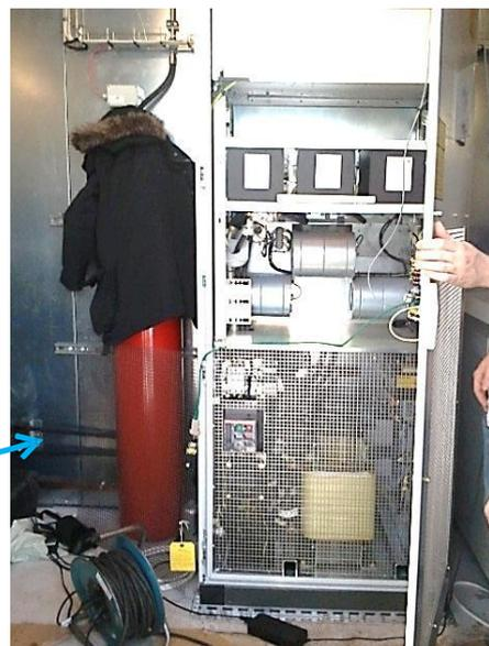
**Figure 19** High AC magnetic field values near the “DC cables” in the control room.
