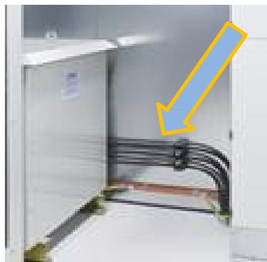
**Figure 23** Up to  $402 \mu\text{T}$  are produced near the cables connecting the AC incoming switchgear (right) with the coupling transformer (left).
