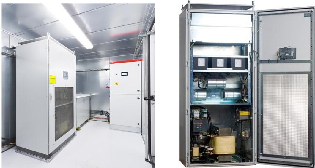
**Figure 4** Control room (left) and detail of the converter panel (right).
