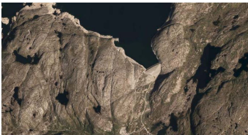
Figur 11. Svartevatn dam located at 59.13, 6.90 in the upper Sira catchment, Norway. Source NVE Atlas, atlas.nve.no, 2015.
