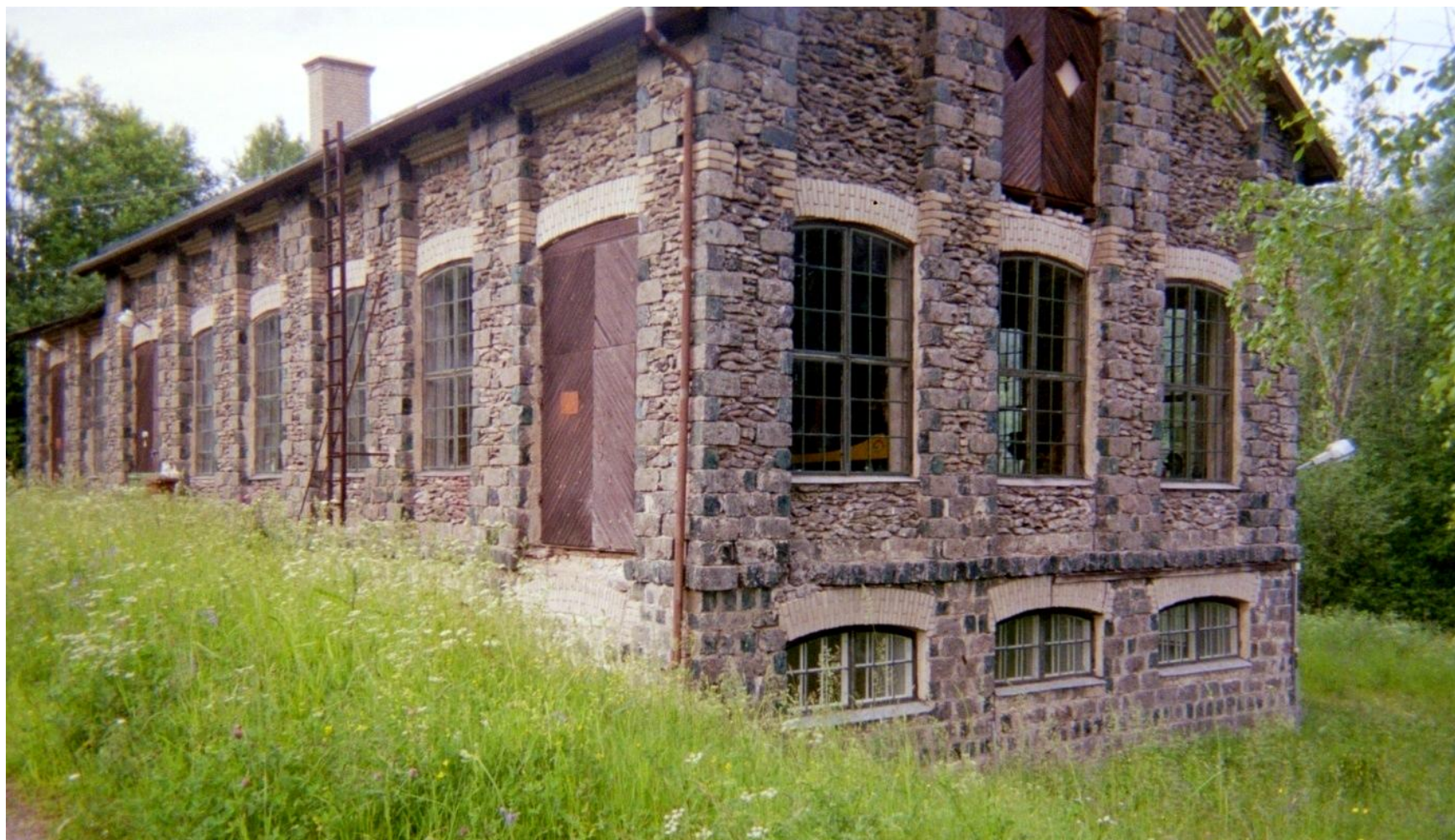
Figure 2. Example of historical utilisation of blast furnace slag (from iron ore reduction). House built using moulded blocks. Please note that the slag blocks were used at the most exposed parts of the building, thus indicating an excellent resistance to weathering.
